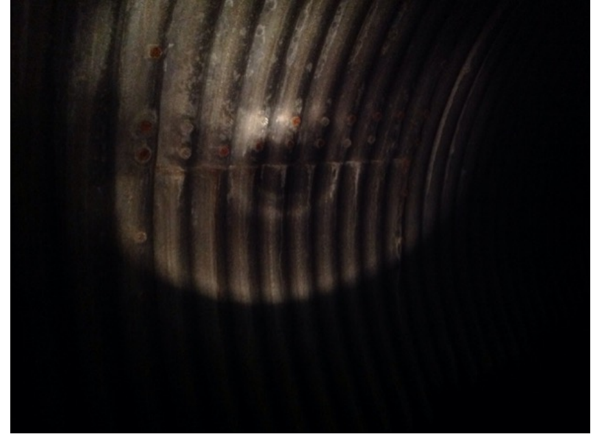
middle section of left culvert is a multiplate - coupled at both ends to CSP
